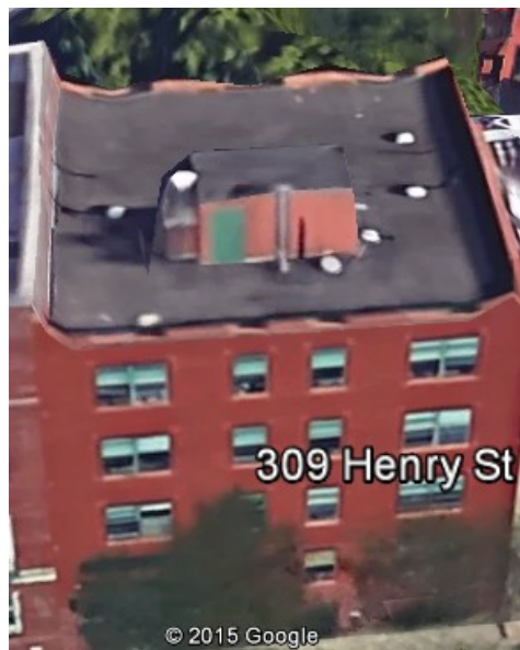
Figure 3 - Aerial view of 309 Henry Street roof via Google Earth.
